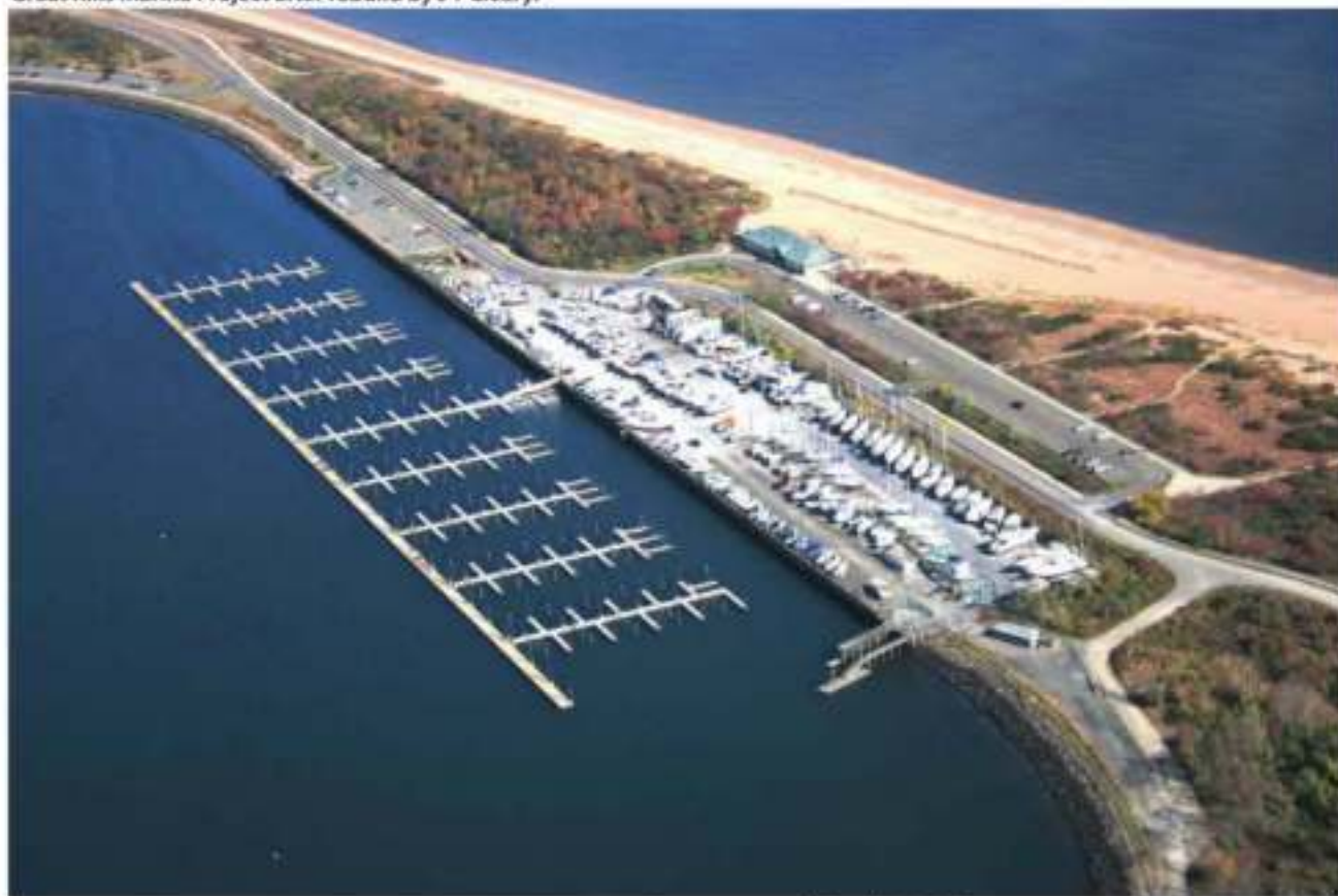
Great Kills Marina Project after rebuild by JT Cleary.
