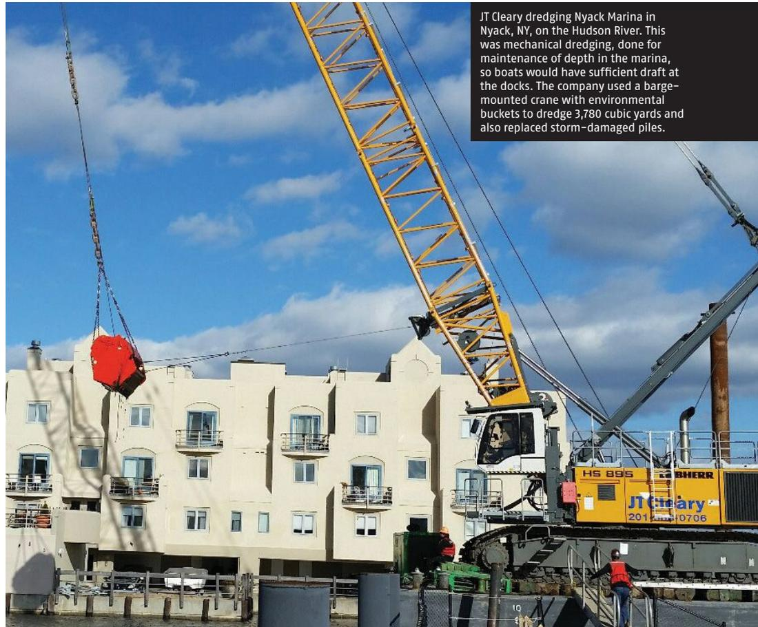
JT Cleary dredging Nyack Marina in Nyack, NY, on the Hudson River. This was mechanical dredging, done for maintenance of depth in the marina, so boats would have sufficient draft at the docks. The company used a barge-mounted crane with environmental buckets to dredge 3,780 cubic yards and also replaced storm-damaged piles.
